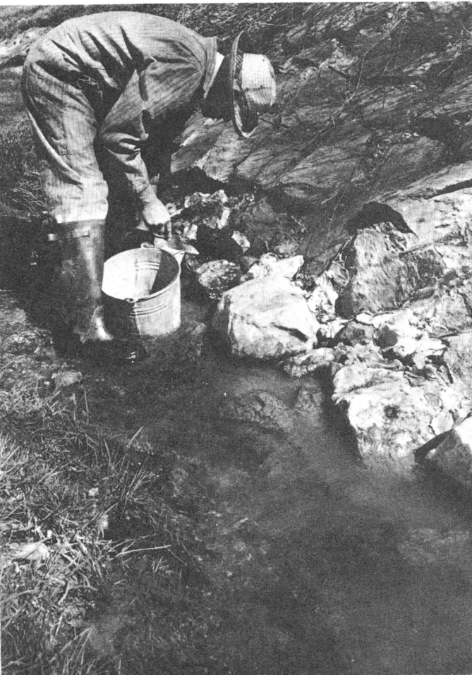
Arming the creek bank with rock.
